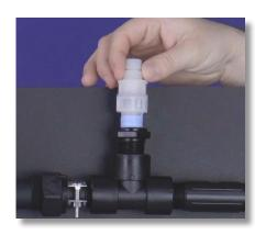
**Step 16:** Install and hand tighten the injection valve into the installation saddle or tee in the supply line. Do not overtighten.
