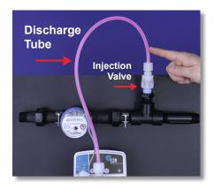
**Step 60:** Chemical should now go up the discharge tube and into the injection valve.
