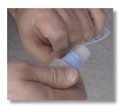
**Step 15:** Take the thread seal tape and wrap it around the threads of the injection valve for the necessary size; either 3/8 or 1/2 inch.
